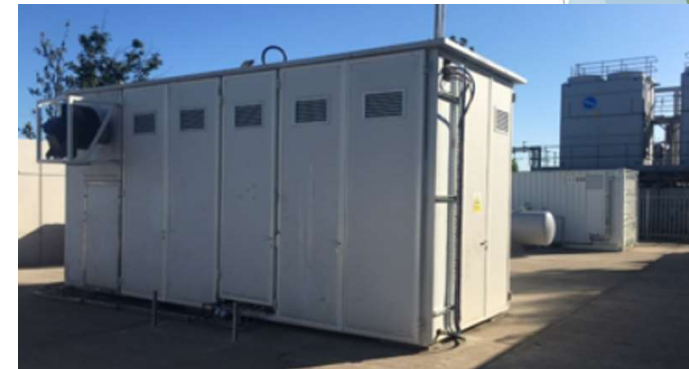
50 m 3 /h hydrogen production system, manufactured by Helbio
